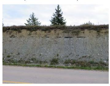
Figure 7: Roadcut Along CO 513 Looking East. Note Gray Bill's Creek Shale Overlain by Tan Stonington Limestone. Photo by Dave Adler.
